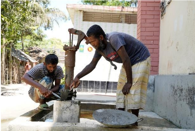
SafePani mechanics fixing school pump.
